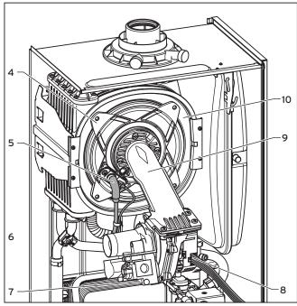
Fig. 7.6 Refitting the burner module
