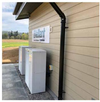
The use of the Vaillant heat exchanger module also contributed to cost savings in the form of saving on glycol required for the heating system. The system is complemented by the Vaillant VRC 700 weather compensating system control which intelligently communicates with all Vaillant appliances.
