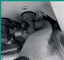
Step 6: open the drain valve until you hear air enter
