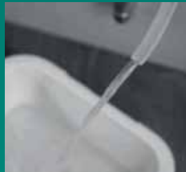
Step 7: open the drain point fully to drain the boiler
