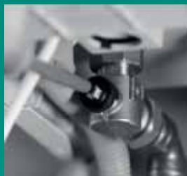
Step 4: close the flow, return and inlet valves
