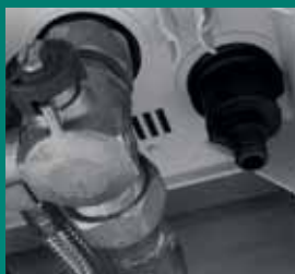
Step 1: locate the drain point beneath the boiler
